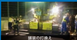
舗装の打換え
